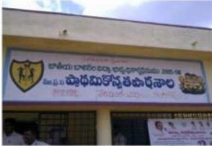
Front View of School building ↑
